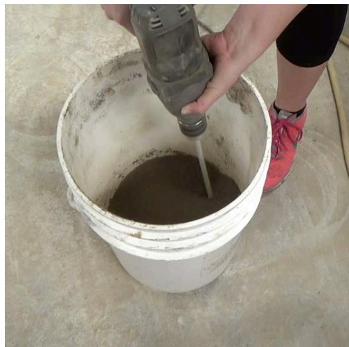
Figure 3-1: Power mixing of soil-cement mixture
